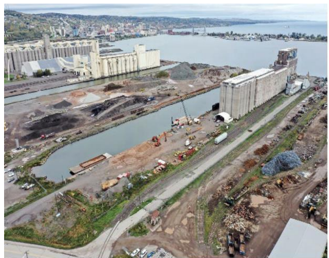
Figure 4: Duluth Lake Port Facility
